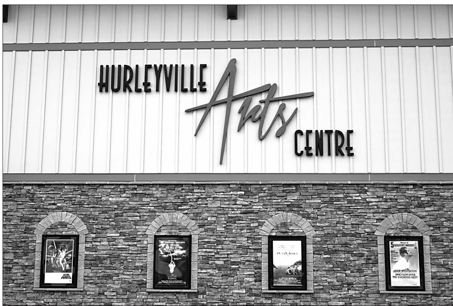
The striking façade of the soon to open Hurleyville Arts Centre on the corner of Main Street and Railroad Avenue.
