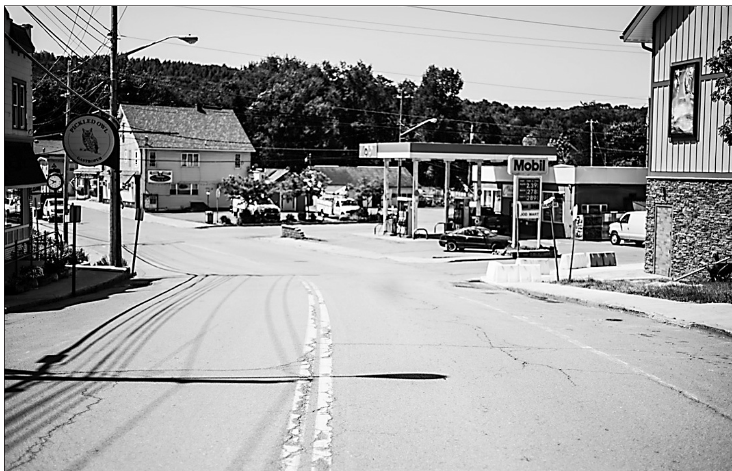
With an increase in pedestrian traffic due to the new businesses located there, Main Street will soon be getting a three-light traffic signal.
